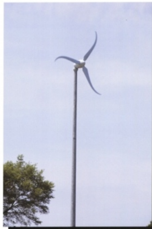
Muskegon's MAREC is home to a wind turbine
