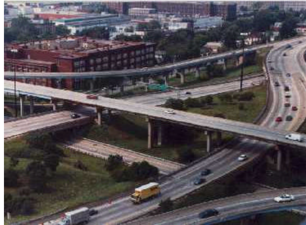
Impervious surfaces within a watershed decrease the amount of land surface area capable of infiltrating stormwater runoff . As a result of increased imperviousness, runoff during a rain event will increase in volume and frequency of flows.
