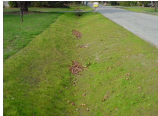
Open channels are another kind of treatment practice used for stormwater. The channels and swales are designed to detain and promote infiltration of stormwater runoff into the soil.
