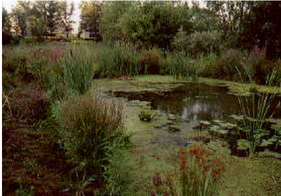
Stormwater ponds are one kind of treatment practice for stormwater runoff . These ponds remove nutrients and other pollutants that are carried in stormwater runoff .
