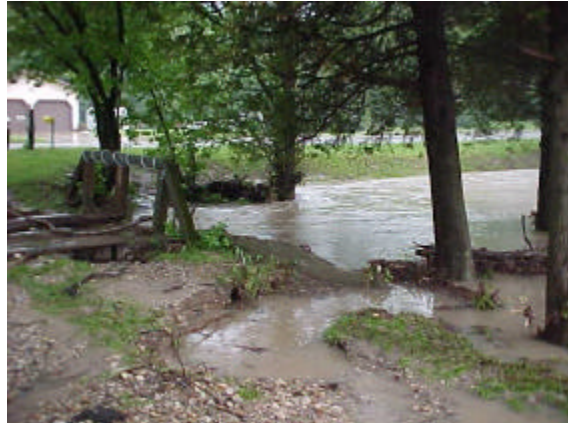
When drainage system capacities are exceeded, surface flooding occurs.
