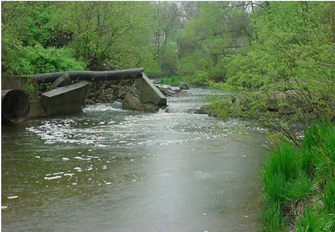
Figure 2: Failed dam below Leonard Street, May 2002
