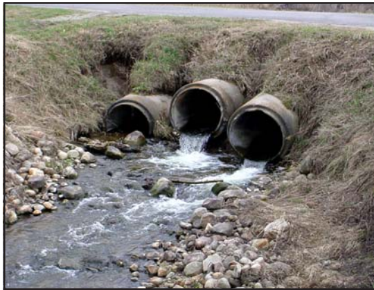
These culverts were broken and partly blocked.
