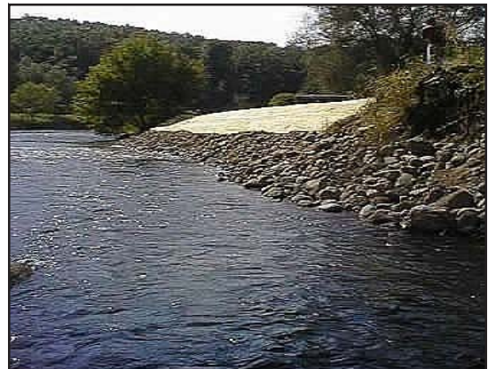
The river bank was graded and stabilized with rip rap and seeded.
