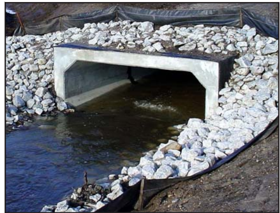
The three cement culverts were replaced with a box culvert allowing the stream to flow freely.
