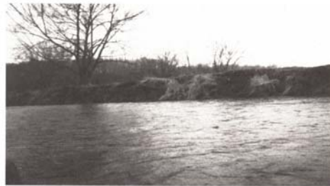
The West Michigan Trout Unlimited is currently working on site plans to stabilize this streambank.
