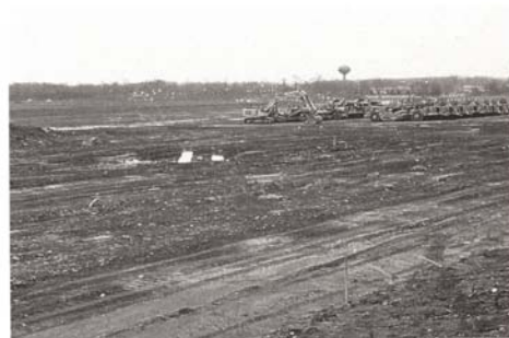
Land is cleared to make room for new development.
