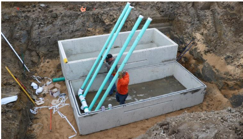
Figure 3. Inlet pipes being laid in the bottom of an iron slag filter. Drainage water enters at the bottom, moves up through the iron slag material (not yet installed) and leaves out a pipe near the top (not pictured) that leads to a nearby surface drain (not pictured). Photo credit: Macatawa Area Coordinating Council.
