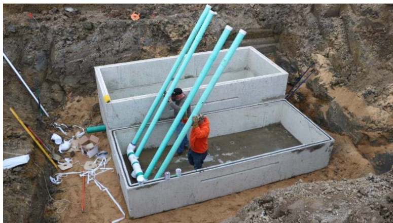
Figure 2. Inlet pipes being laid in the bottom of an iron slag filter. Drainage water enters at the bottom, moves up through the iron slag material (not yet installed) and leaves out a pipe near the top (not pictured) that leads to a nearby surface drain (not pictured). Photo credit: Macatawa Area Coordinating Council.
