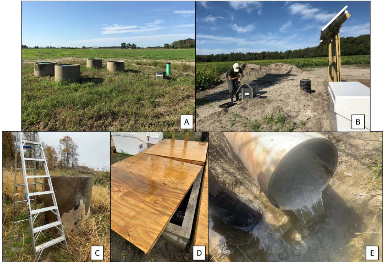
Figure 4. Photos of different sampling locations. A) Behind Mill 1 with completed iron slag filters in place. The green tube (far right) is an inflow sampling port that was installed only at this location. Access ports (for cement upright tubes) are for two slag filter basins (considered to be one slag filter site) that receive tile drain water from the adjoining field (in background) and are used to sample outflow. B) Research Assistant, Emily Kindervater, using a hand pump siphon to sample from a below-ground control box (inflow) at Fillmore Flex; Oak Grove 2 has a similar constructed inflow access (not shown). C) Slag filter outflow access point for Oak Grove 2, which required a ladder to remove the large plastic cap to sample outflow water. D) Slag filter outflow access point at Fillmore Flex, which is covered with large plywood lids. E) Outflow pipe at Behind Mill 1 directly after installation; the white particulate residue inside the tube is from the calcium carbonate layer placed on top of the iron slag inside the tanks to balance pH.
