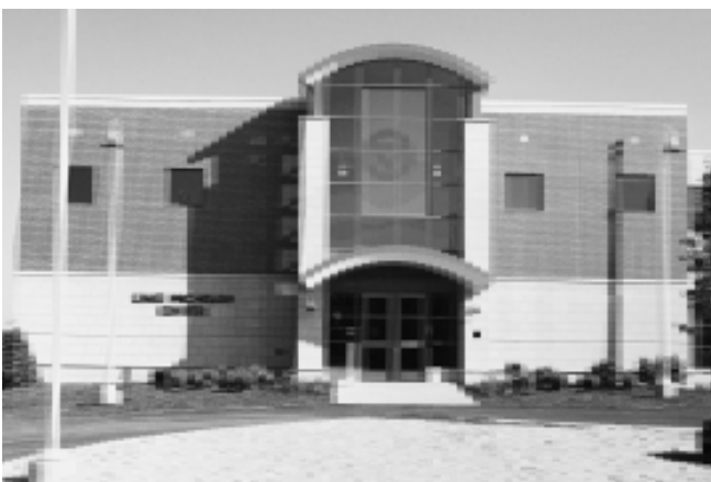
AWRI's new Lake Michigan Center was dedicated in June.
