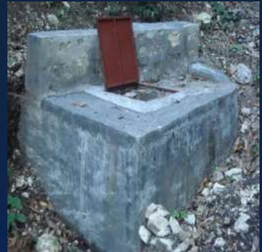
Concrete spring capping
