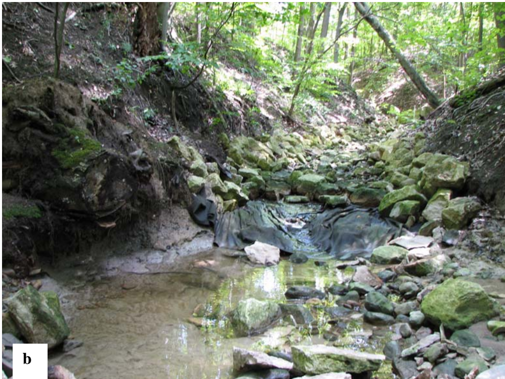
Fig 19 a) Boulder armoring newly installed in the Little Mac ravine. Photo taken by P. Videtich, 09/03/2002. b) Boulder armoring failure in Little Mac ravine. Photo taken by P. Womble, 07/20/2006.
