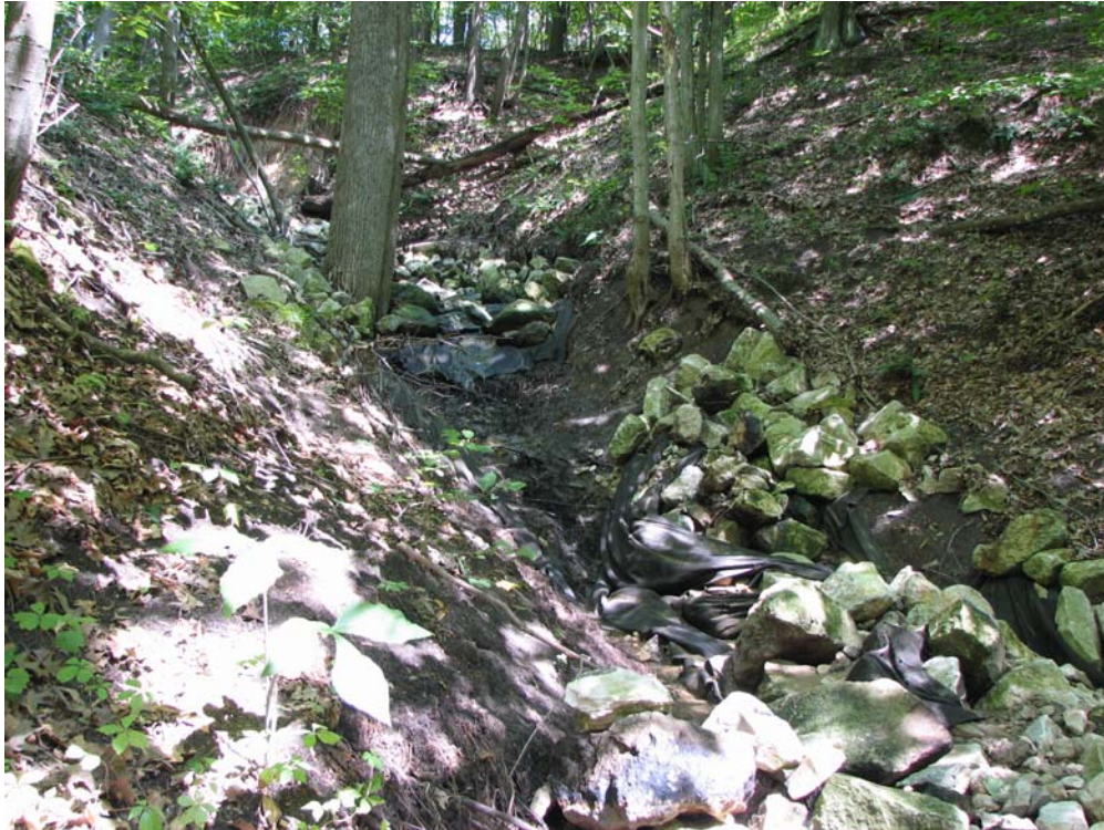
Fig 20 Boulder armoring failure and underlying blanket mobilization in a ravine tributary just south of the Calder Art Center. Photo taken by T. LaCross, 08/01/2006.
