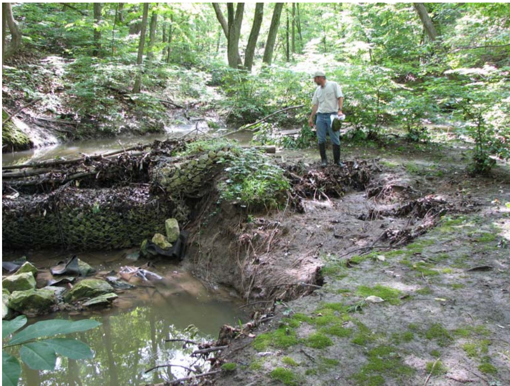
Fig 21 Lowest check dam in the Little Mac ravine showing increased erosion due to the stream bypassing it during high flow conditions. Photo taken by P. Womble, 07/20/2006.
