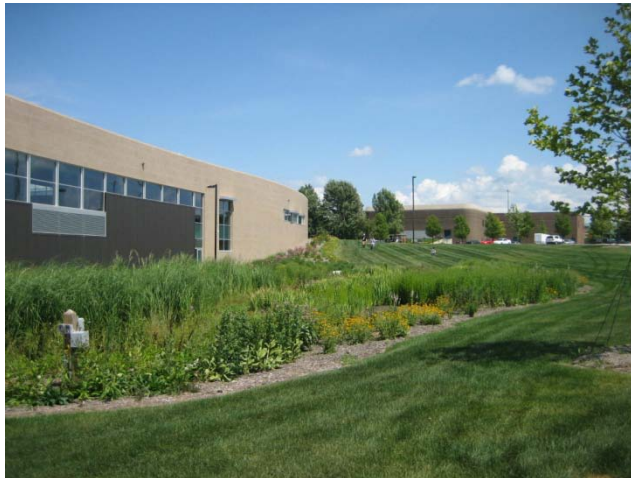
RAIN GARDEN – LAKER TURF BUILDING
