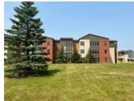
Existing South Living Centers
