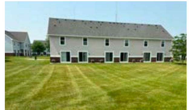
Existing Conditions: Exterior of Laker Village
