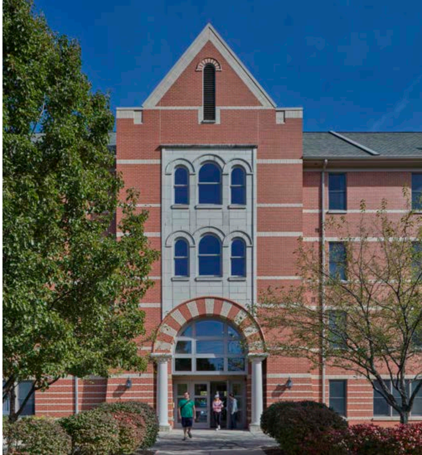
Existing Winter Hall
