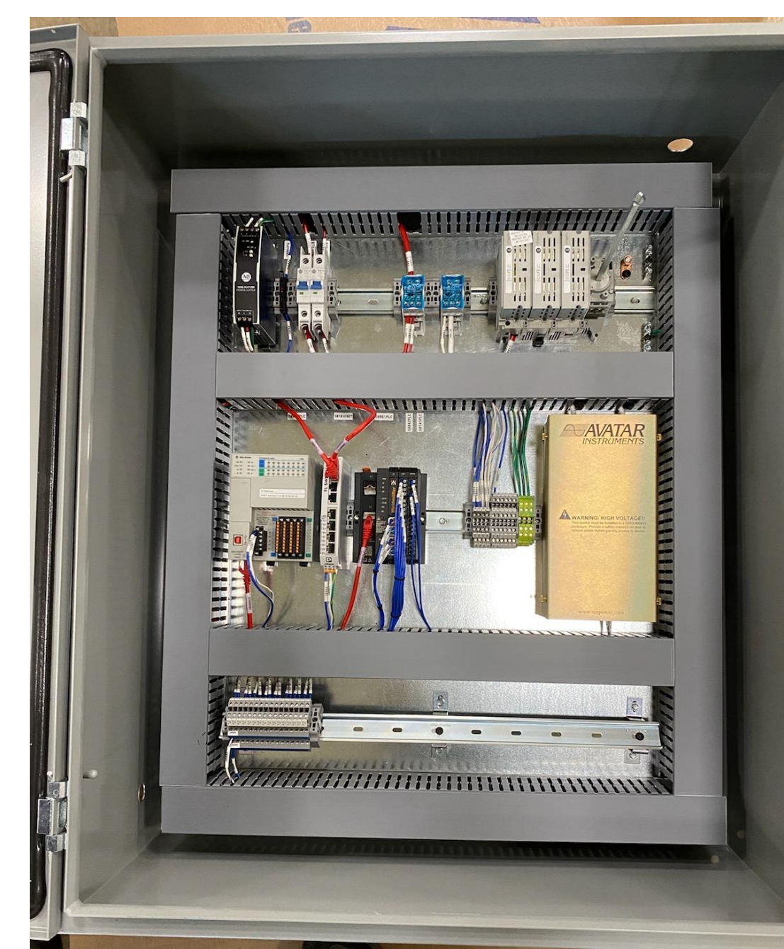
Electrical Panel Build
