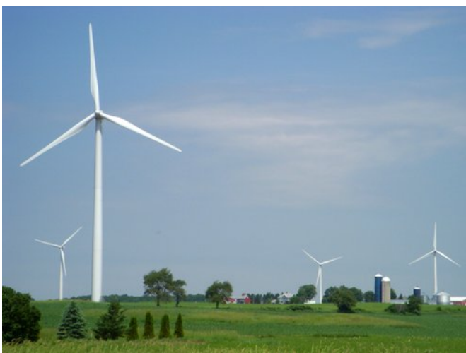
Figure 2a. Wind farm in Wisconsin with 86 turbines each at 1.5 MW capacity (Forward Wind Energy Center, 2009). (US Dept of Energy – NREL)
