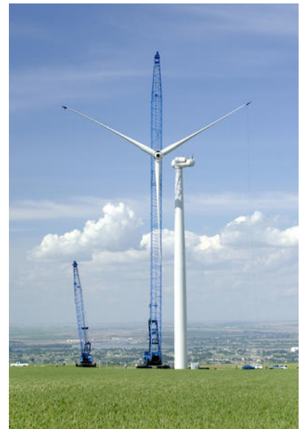
4c. Installing the blades for a 1.3 MW turbine at the Nine Canyon Wind Project (Washington, 2002).
