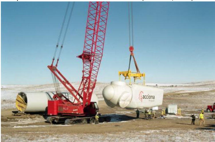
4b. Lifting the 163,000 lb. nacelle and rotor hub for a 1.5 MW turbine at Tatanka Wind Energy (North Dakota, 2007).
