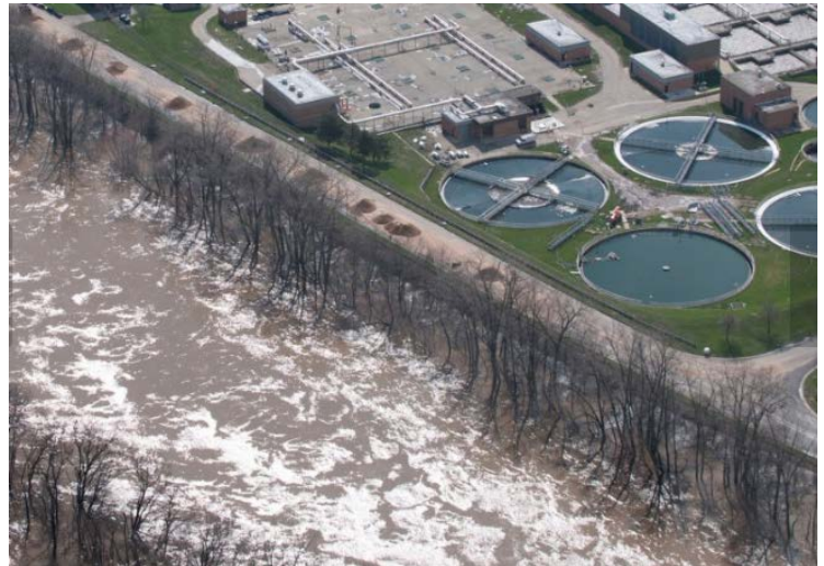
Grand Rapids Water Resource Recovery Facility
