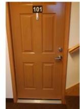
New beveled threshold and lever handle installed to make unit entry accessible
