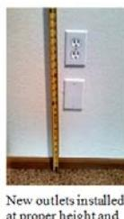
New outlets installed at proper height and old ones capped off
